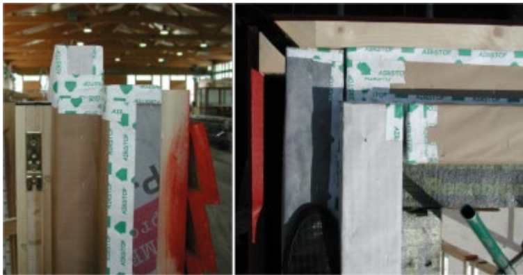
Figure 55: External wall corner: on the left, prefabrication (view); on the right, assembly (top view)
