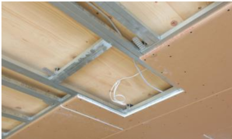
Figure 41: Floor system with whip arm and GKF with good sound protection properties, source: Knauf company
