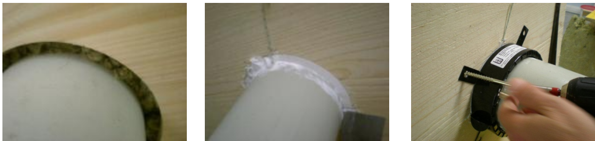
Figure 87: Installation of a fire protection collar directly in an unclad solid timber wall; left: Filling up the annular gap, center: intumescent fire protection compound, right: fastening of the fire protection collar
