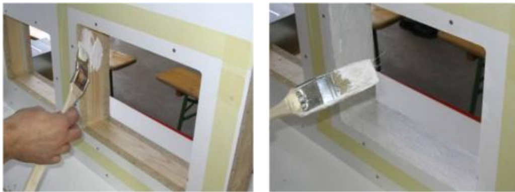
Figure 84: Application of coating on reveal and reveal coating, source: Würth company
