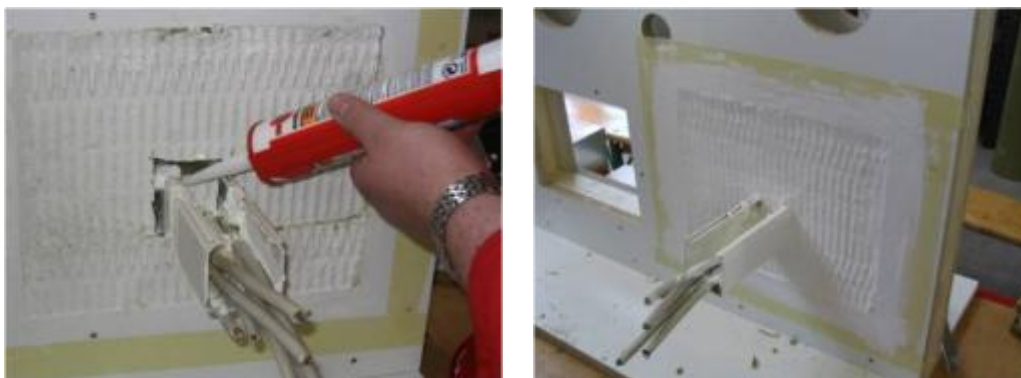
Figure 86: Sealing of cable penetrations and finished partitioning, source: Würth company
