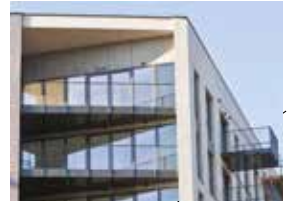
Bridport House, London 8 storeys: The highest building in London built using CLT was erected in only 12 weeks.
