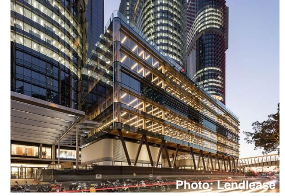
International House Sydney, Australia
